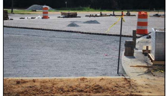
Delta Hall's Parking Lot Under Construction
